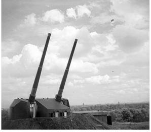
In January 1941 a more powerful anti-aircraft gun was requested by the War Office and the 5.25 Naval gun was chosen, the first guns were completed in 1943. There were two separate mountings for the gun, the Mk IA solely for anti-aircraft use and the Mk IB for a dual anti-aircraft/Coastal defence, these had an armoured turret. The guns were first installed in the London area and naval bases such as Plymouth and Portsmouth.
