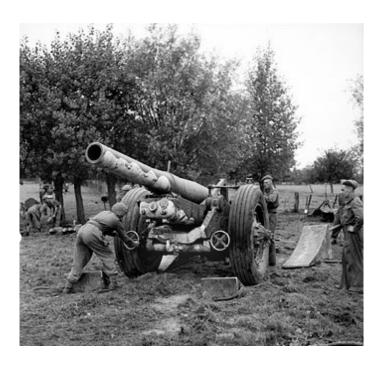
After Dunkirk there was a great shortage of heavy artillery so requests for a weapon of around 8" in calibre with greater range than the current 8" Howitzer were made. Firing trails were conducted to see how much stress the 8" Howitzer carriage could take and so it was decided to develop a 7.2" weapon that fired a 200lb shell at 1,700fps. Barrel liners of existing 8" weapons were replaced by a 7.2" liner
